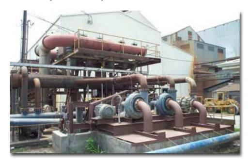
A sugar cane factory in Jeanerette, Louisiana, was experiencing difficulties and equipment failures due to excessive abrasives (sand, grit, small rocks) introduced during the initial washing phase.
